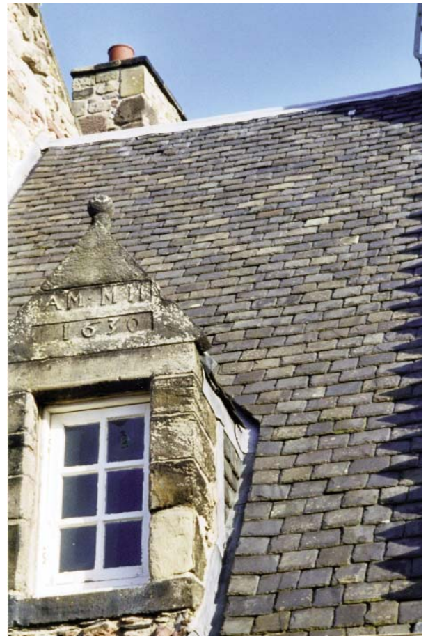
Traditional Scottish Slate Roof, Edinburgh, Scotland
