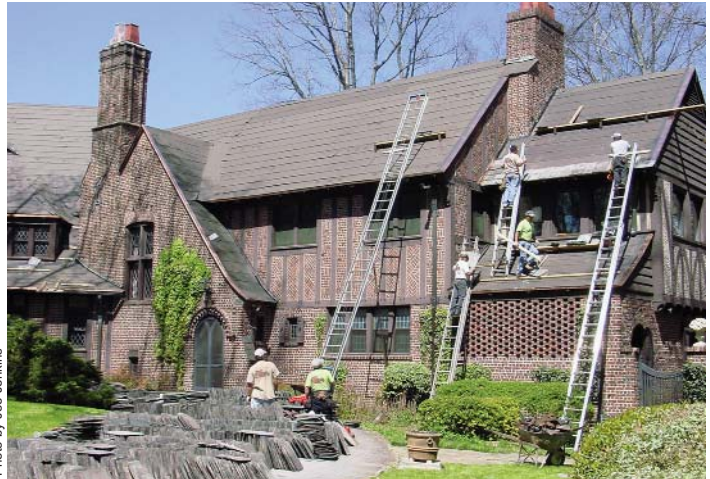
Glenridge Hall, front entrance, after the original slate had been removed and stacked in the driveway and the new felt installed. Re-slating is just beginning.
