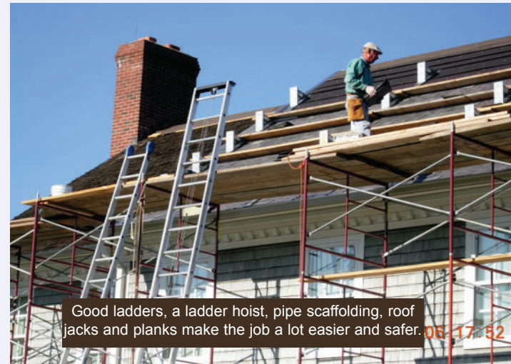
Al's Solid board sheathing makes a perfect deck for a slate roof.
