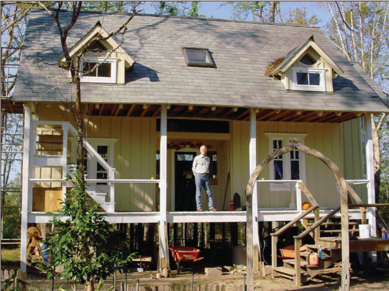
"It's not rocket science," Dave tells us. His handiwork included a band of hand-rounded slates across the roof, flashing around dormers and skylights, plus ceramic tile ridges. The force of the winds that battered his home is evident in the photo below, which shows only one of the many tress that succumbed to Katrina's massive assault.
