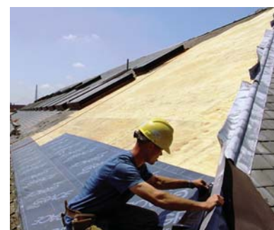
Figure 4: Traditional slate roofing systems, despite their incredibly successful performance, are being largely abandoned in favor of plywood roofs with peel and stick underlayment.
