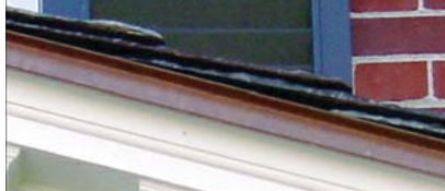
Figure 6 (above): No slate lies flat on a slate roof. Every slate is angled, which is why they should not be walked upon and why the starter course requires a cant.
