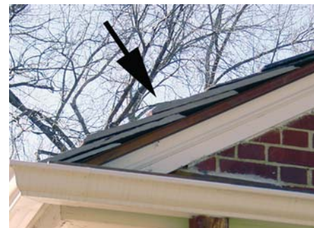
Figure 33: Diamond blades cut a square edge on slates, making them stick out like a sore thumb.
