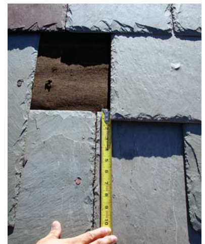
Figure 9 (above): Headlap is a critical detail on a slate roof. Lack of headlap will cause an entire roof to be condemned. Read more about headlap in TR6.
