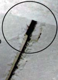
Figure 11: When the slate courses are spread too far apart vertically, negative headlap can result, creating holes all through the roof.
