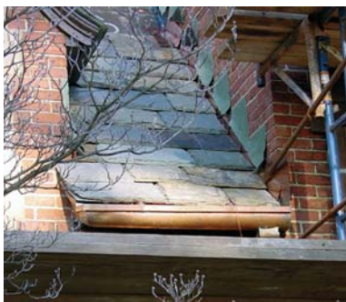
Figure 31: This gutter is just waiting for a snow avalanche to knock it off.
