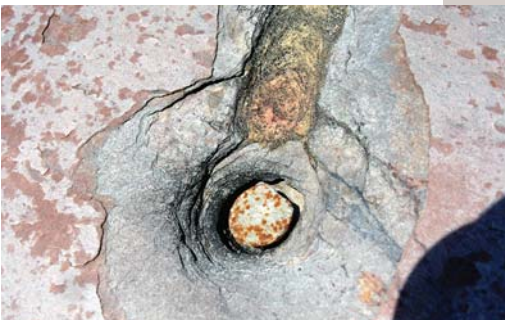
Figure 15: A protruding nail head eventually wears a hole in the overlying slate.
