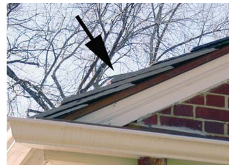
Figure 33: Diamond blades cut a square edge on slates, making them stick out like a sore thumb.
