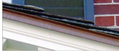
Figure 6 (above): No slate lies flat on a slate roof. Every slate is angled, which is why they should not be walked upon and why the starter course requires a cant.
