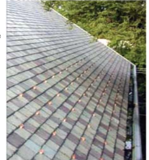
Type SGAR-SLS for retrofit on slate
