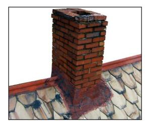
henever it's raining and someone sees evidence of water leaking, the first thing they think of is a roof leak — and they are probably right. However, it can also be a masonry leak. If the leak shows up next to a brick chimney or at an opening in a masonry wall and the flashings above the area are installed properly and in good condition, the masonry is probably the problem.
