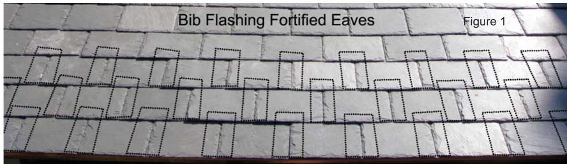
Each bib is at least 6" wide and slid up underneath the slates until they hit the slating nails.
