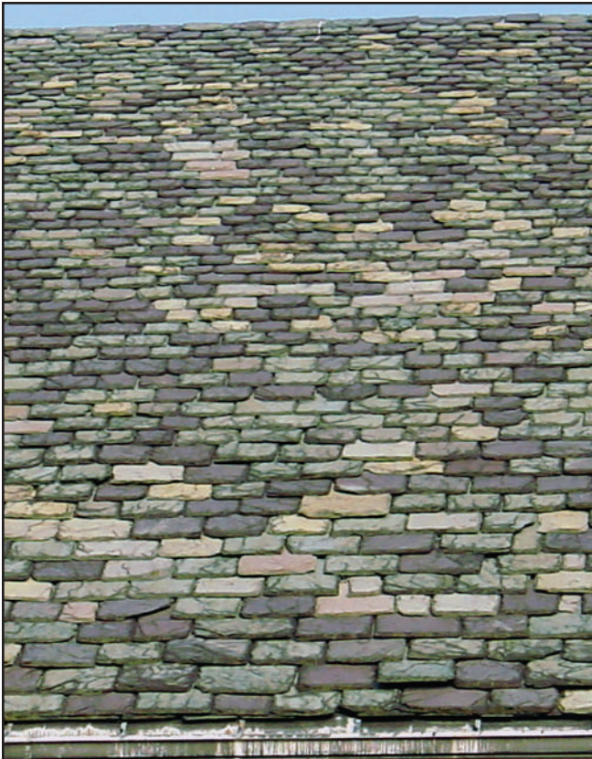
Figure 6: Graduated slate roof. Slates vary in both widths and lengths. This roof also blends several colors of slate.
