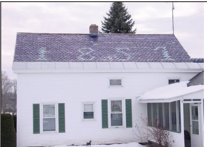
Figure 2: Vermont purple slate with a Vermont unfading green slate date, located near Fair Haven, VT. At 152 years of age this roof could still function admirably for generations.
