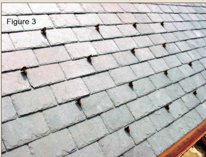
This VT unfading gray slate roof was installed with 4" headlap along the bottom three feet of the eaves (bottom 5 courses), while the remaining field slates have 3" headlap. The difference in exposure is not detectable by eye. This is the correct way to fortify the eaves on a slate roof when ice-damming is a concern. Underlayments do not work in the long run.
