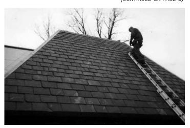
Putting the finishing touches on one side of garage, Erie, PA. Most of the faces had hips on both sides so we started in the middles and worked our way to the edges. Note how the steep roof pitch allowed us to lay ground ladders right on the roof, thereby avoiding the need for any roof planks.
