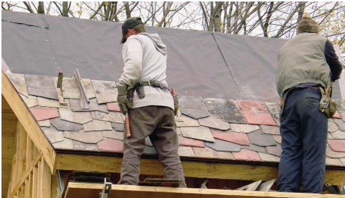
Figure 9: Ragged butt style of slating on a bat house at Slippery Rock Univ., Slippery Rock, Pennsylvania (see back cover). In this case, three lengths of slates are being used (16", 18" and 20"). The tops of the slates are lined up with chalk lines spaced for 16" slates and allowing for a three inch headlap (a chalk line every 6.5"). The longer slates are allowed to hang down, but are trimmed off to leave a "battered" or "ragged" effect.
