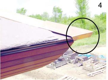
3) Start with a piece of flashing at the bottom of the hip, cut at an angle to match the roof contour. 4) The flashing should be folded at the bottom to cover the end of the nailers. This is 20 ounce copper, but a lighter gauge is suitable.
