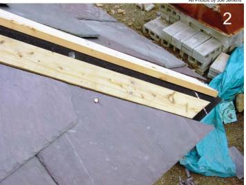
1) Nail or screw furring strips to both sides of the hip or ridge. The thickness of the strips must be 3x the thickness of the slate. 2) Install the slate in the field of the roof right up against the wood nailers. Always use two nails per slate.
