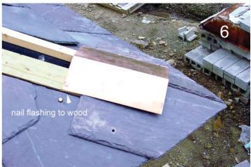
5) Install the first pair of slates over the flashing, also cut at an angle. 6) Install the second piece of flashing.
