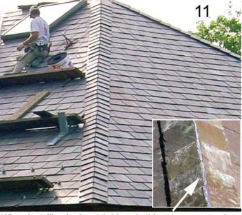
When installing horizontal ridges in this manner, a good quality caulking seal at the ridge is recommended.
