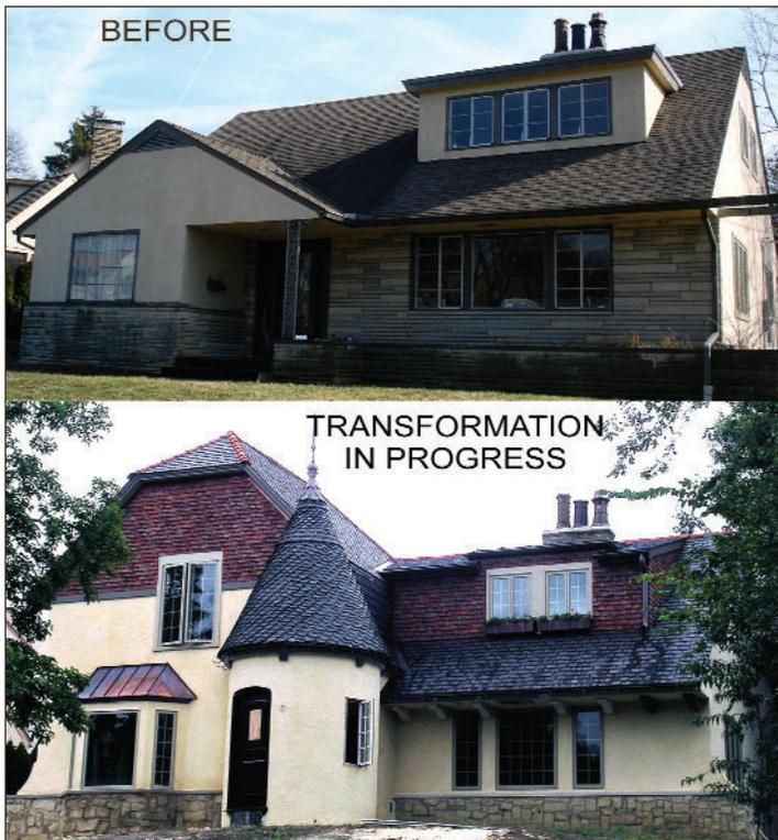
and the second floor was extended to provide additional living space. A new turret entry was built, and an original design was created for installing the slate on this roof. Salvaged Virginia Buckingham slate was installed on the roof, while a veneer was installed just above the foundation and French tile was installed on the exterior wall of the upper floor.
