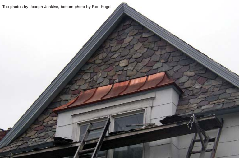
▲ A slope transition on a roof plane often requires a transition flashing, sometimes called an "apron." The flashing is folded with a Z bend to compensate for the angle of the slate on the upper half (making a cant strip unnecessary), and is nailed along the top edge, then held down along the lower edge with cleats, as shown. Dimensions vary, but 16", 20 ounce copper stock is shown used above. ▼ Unique slate siding and copper roofing installed by SRCA member Ron Kugel of Evans City, PA.
