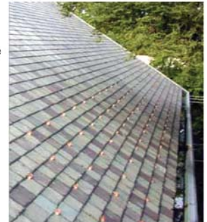
Type SGAR-SLS for retrofit on slate
