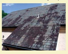
determine there is a forced venting of moisture through the roof at this location.....also note the crisp line of the juncture and that the stain appears to "run" downhill from it. Also note a little further up the roof there appears to be a de-
