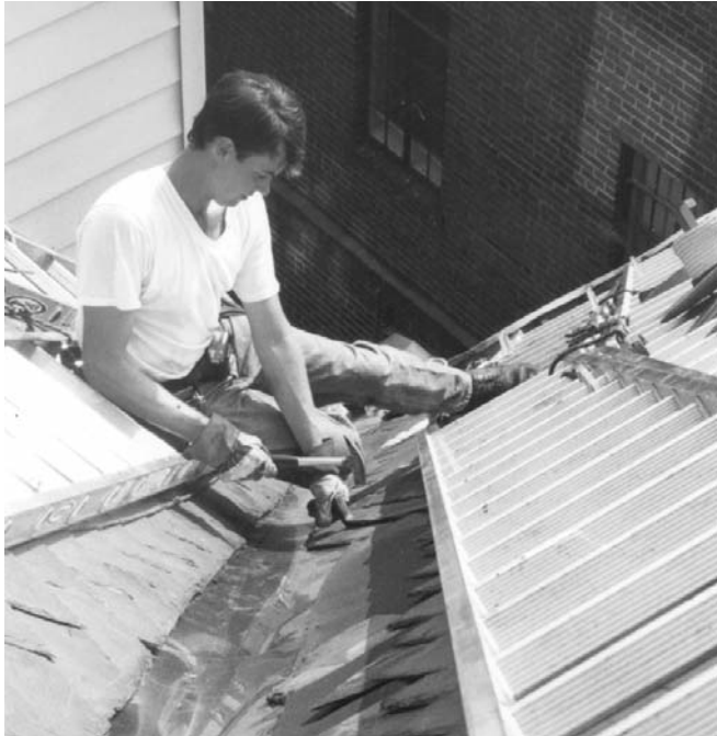
Stacy Moore replacing a valley with copper on the First Presbyterian Church in Greenville, SC.
